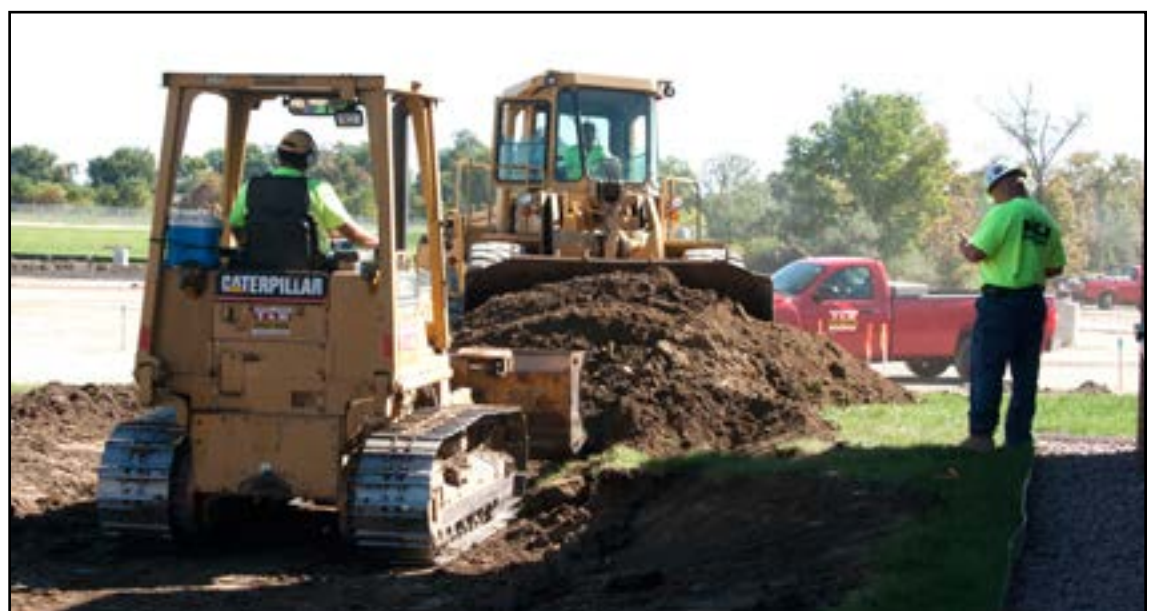
(Bottom) Construction workers continue to clear land where an additional parking lot will be constructed. This lot will provide better access for students to park closer to their classes. (Top Middle) An aerial view of the development of the new road running behind the Applied Science, Biomedical Technology Center, and the Fitness Center.
