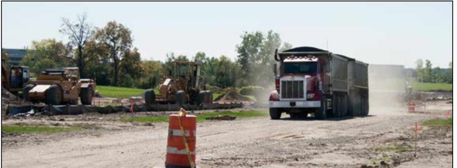
A semi-trailer hauls debris down the future site of the new road that will connect 6 Mile to 7 Mile Roads. Vehicles will be able to travel around the perimeter of campus instead of Fox Drive, helping to keep pedestrians safe. PHOTOS BY LINDSEY WELLS
