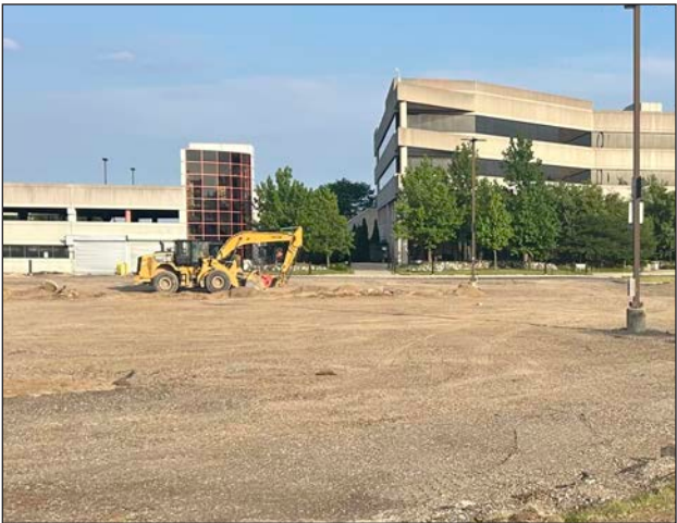
Construction began on the former Comerica Bank Property in late summer 2025. Whole Foods and many other retailers will soon line the corner of 6 Mile & Haggerty in the year to come. (Photo Courtesy of Livonia-Westland Chamber of Commerce).
